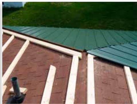
space between the existing shingles and your new roof which forms an insulating thermal and vapor barrier.
